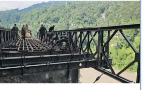
RNS I Gangtok: In a remarkable engineering feat, Army engineers constructed a 70-foot Bailey Bridge on the Dikchu-Sanklang road in Sikkim within 72 hours, restoring connectivity that was severed due to recent floods. The construction was undertaken by the Trishakti Corps Army Engineers, commencing on June 23, according to the PRO Defence Guwahati.
